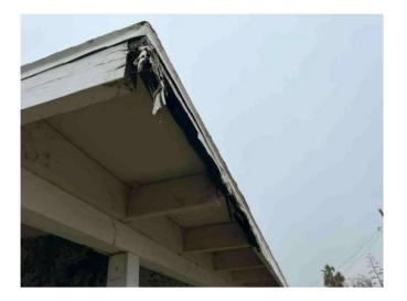
ROTTED WOOD ON THE COVERED PATIO NEEDS TO BE REPLACED AND FRESHLY PAINTED. COST TO CURE WOULD BE \$150 TO \$200.
