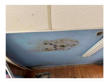
ORGANIC GROWTHLIKE SUBSTANCE ON THE CEILING IN THE SHED COULD BE HARMFUL. CEILING NEEDS TO BE REPAIRED IN THE DETACHED SHED. COST TO CURE WOULD BE \$350 TO \$400.
